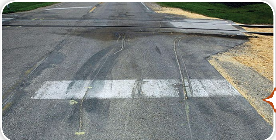
Gouges in the roads and vehicle deformation serve as areas of extreme scrutiny when investigating vehicular accidents.
