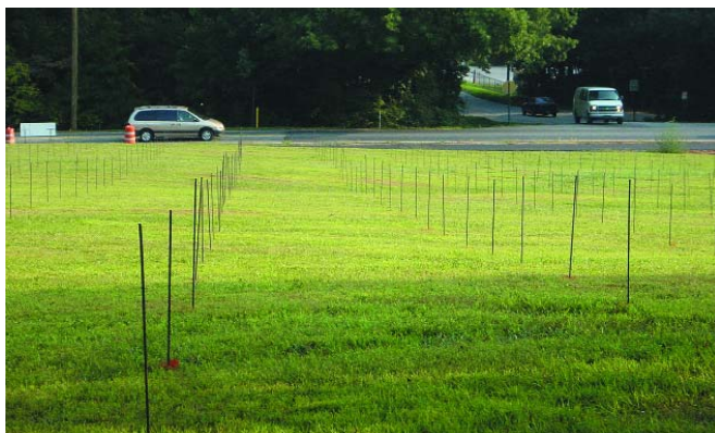
Sections of rebar in place on the grid
